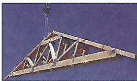
**✓** A single lift point may be used for bundles of top chord pitch trusses up to 45' (13.7 m) and parallel chord trusses up to 30' (9.1 m).
