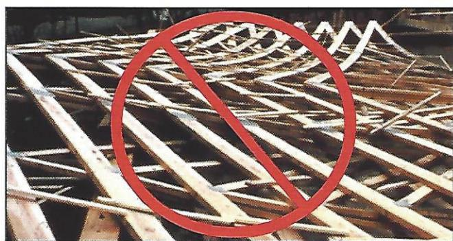
**WARNING** Roof and floor trusses that are not properly braced per BCSI or sheathed are not able to resist lateral impact loads associated with falls. A falling worker attached to an inadequately braced set of trusses could cause all the previously set trusses to collapse in a domino effect.
