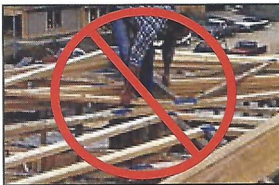
**DANGER** Do not walk on trusses or gable end frames lying flat, they do not have the structural strength to support a worker safely while oriented flat.
